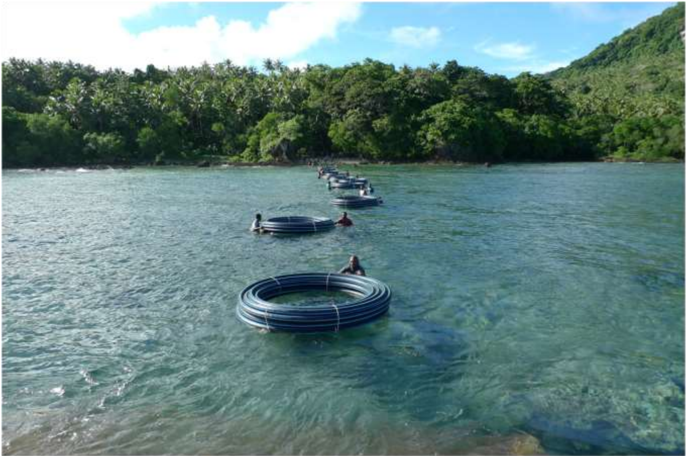
MATERIALS FOR THE GRAVITY-FED WATER SYSTEM ARE DELIVERED TO THE ISLAND OF MOTOLAVA, TORBA PROVINCE.
